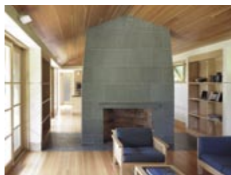
Above and right: The living room fireplace uses a Rumford-style firebox designed to maximize energy efficiency. The chimney and the surrounding stone floor are designed as a thermal flywheel – absorbing heat during the day and re-radiating it at night. All living and sleeping areas open out through large doors to wide porches and the grass-covered central space.
