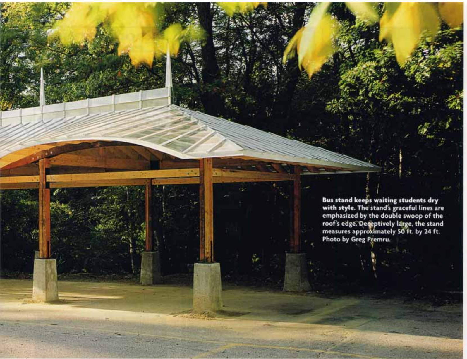
Translucent roof allows the stand to glow at night. Moskow covered the roof with a smooth fiberglass sheathing thin enough to bend easily over the curves. The curved fascia is plastic. Photo by Greg Premru.
